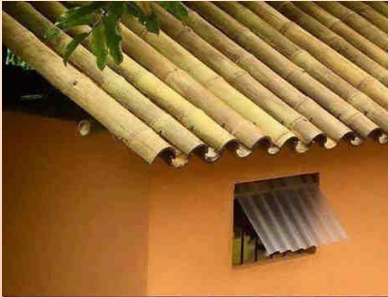
Plate 1: Use of bamboo in roofing as was observed in households adjacent to Udzungwa Mountains, Kilolo District
